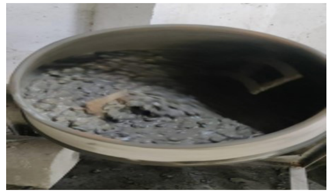
Figure 2: Mixing of concrete.
