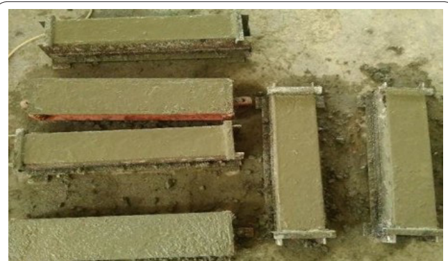
Figure 4: Casting of flexural beams.
