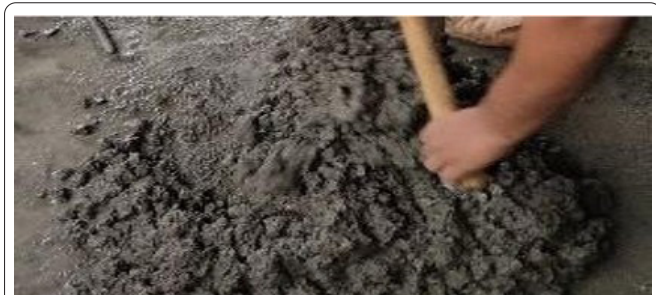
Figure 2: Conventional concrete mixing.
