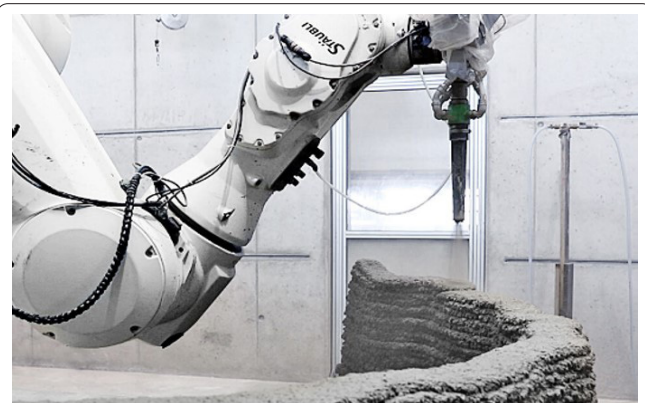
Figure 5: Additive manufacturing based on spaying: SC3DP, ITE, TU Braunschweig.
