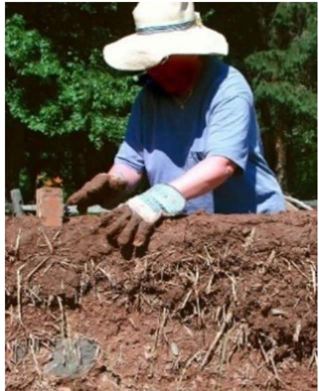
Figure 1: Earthen wall constructed with the Cob technique.
